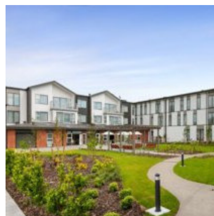
BUPA RETIREMENT VILLAGES NAPIER, TOTARA, CROFTON DOWNS, PALMERSTON NORTH, ASHFIELD
