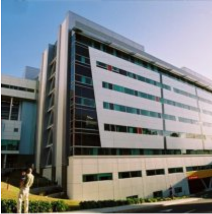
AUCKLAND HOSPITAL AUCKLAND, NEW ZEALAND
